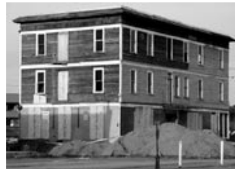
Caribou Hotel, Carcross, undergoing restoration work, 2006 Yukon government photo
