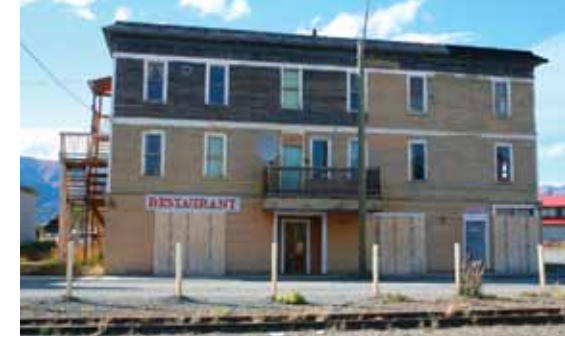
The Caribou Hotel in Carcross was designated as a Yukon Historic Site in 2008. Yukon government photo
